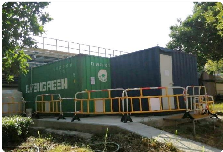
Pilot study at Shatin STW Treatment capacity: 5 m 3 /d
